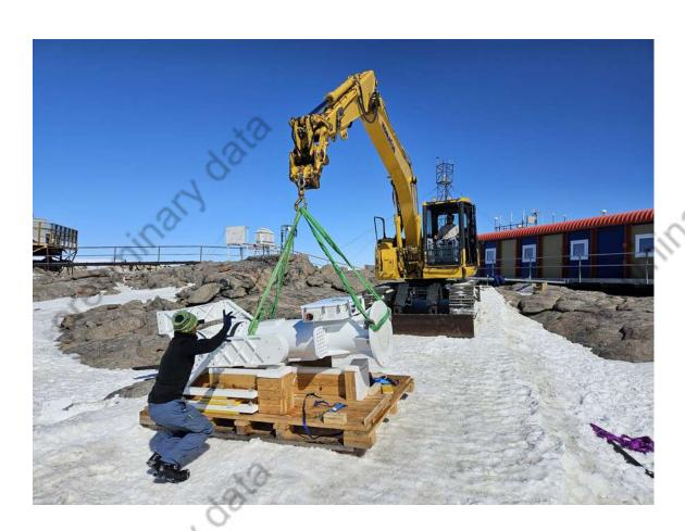
Threaded rods in concrete base prepared in 23/24 did not fit...
